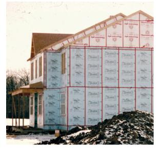
All joints and seams in sheathing sealed with compatible and durable tape
